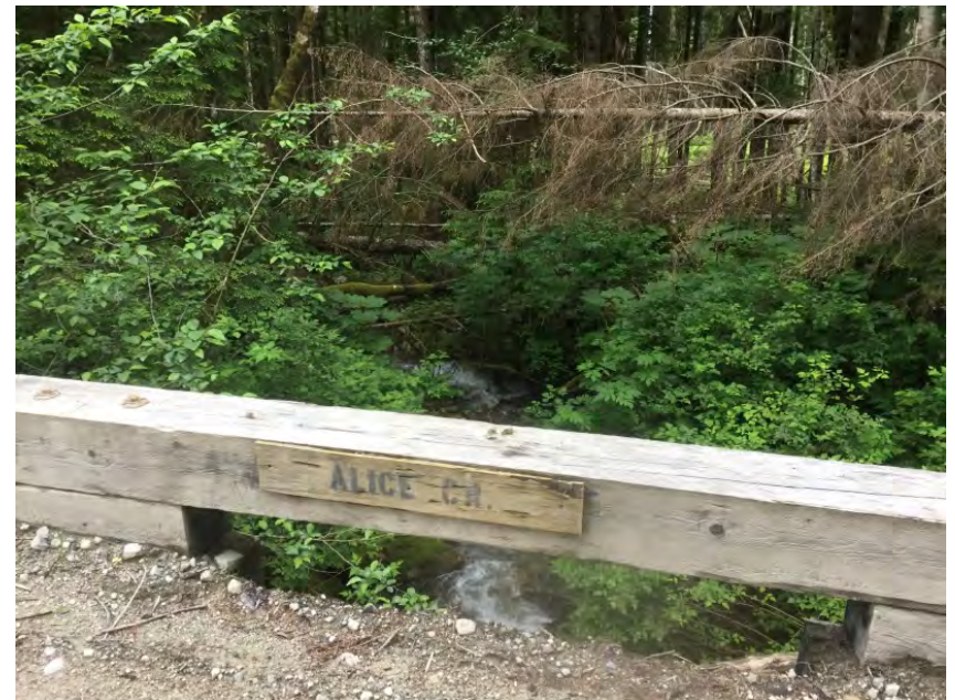
Looking downstream from deck
