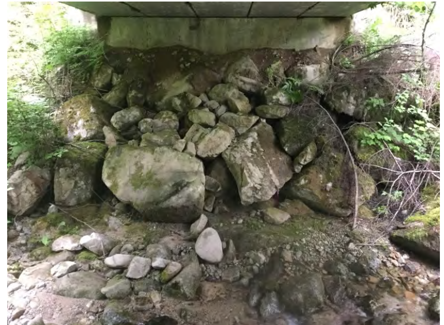
Right Bank Abutment when facing downstream
