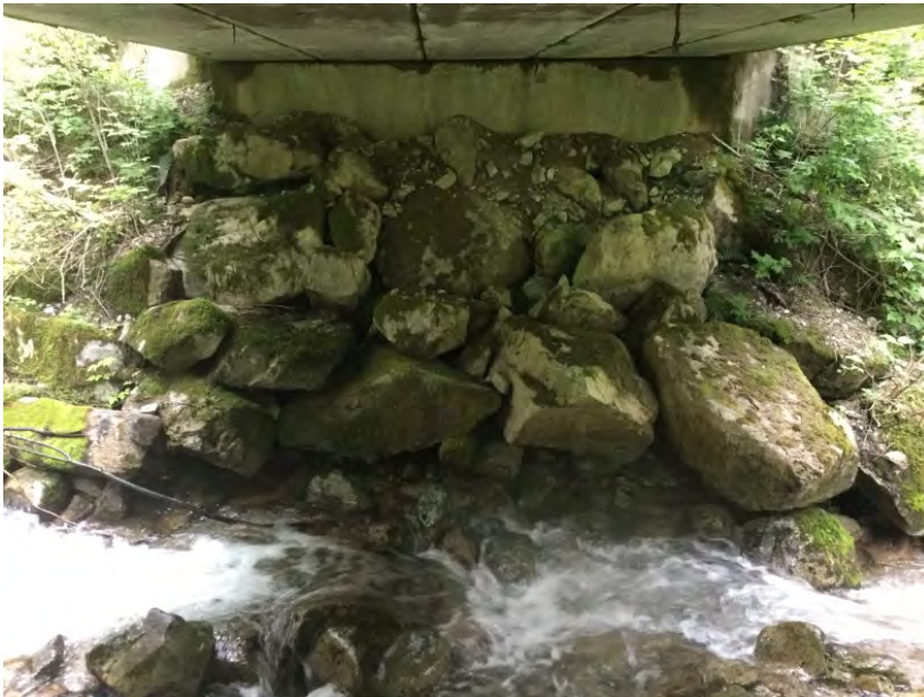
Left Bank Abutment when facing downstream
