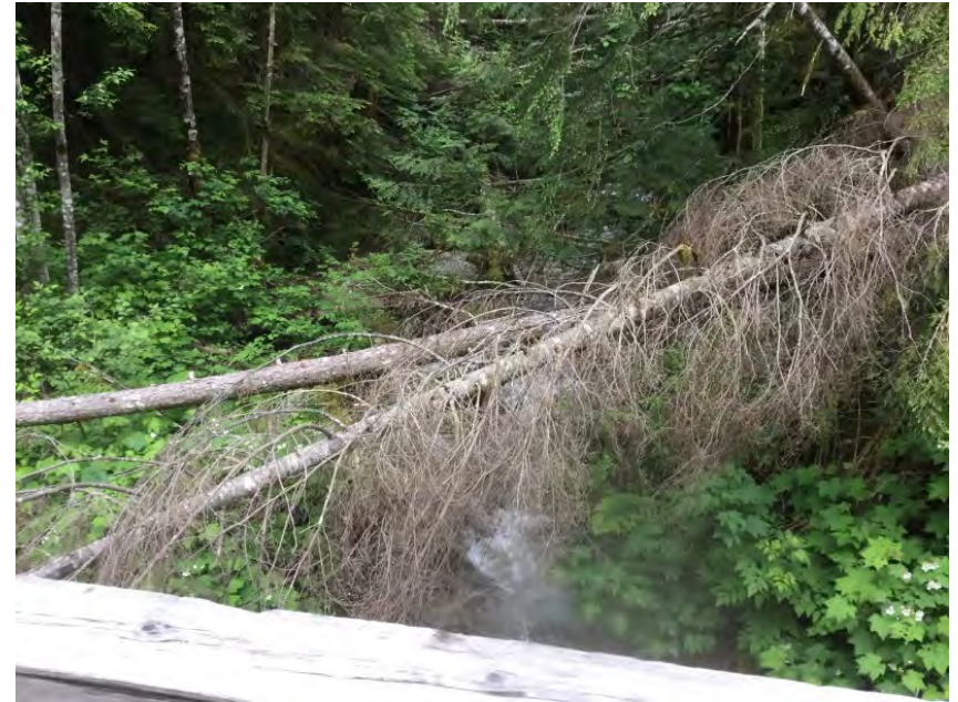
Looking upstream from deck
